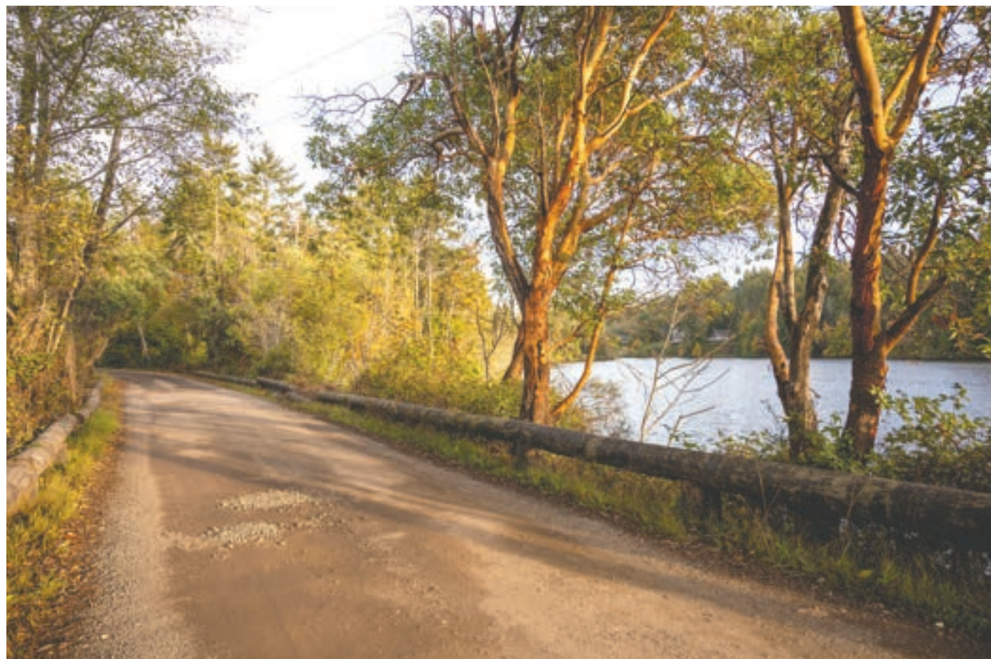
The causeway to YMCA Camp Colman along the cove will see significant changes in 2024. Tina McKail, KP News
